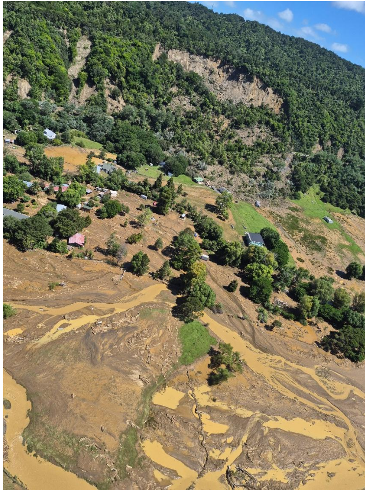
Figure 11: Aerial photograph of flooding in the Hicks Bay area in January 2026.
