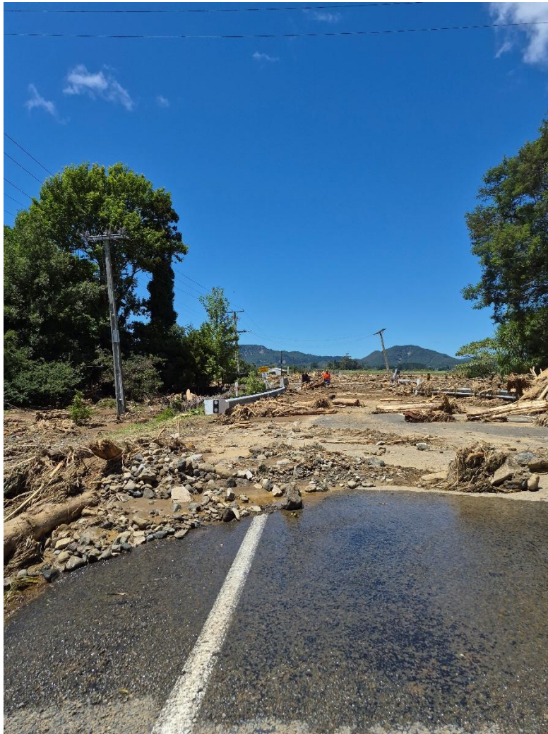
Figure 12: January 2026 major event repair of a pole washout after flood waters receded.
